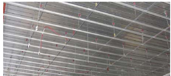
BCA-compliant acoustic ceiling installation in a government building, built from Studco products
