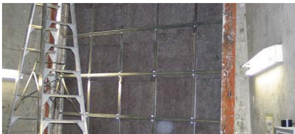
Acoustic testing of Studco wall system using CSR Gyprock plasterboard
