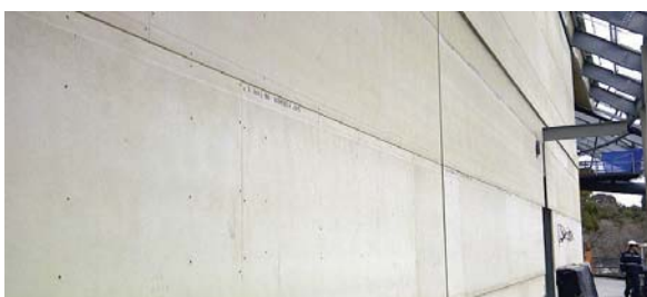
Wall designed for extreme acoustic and impact performance, built from Studco steel stud systems and USG Fibrerock lining boards
