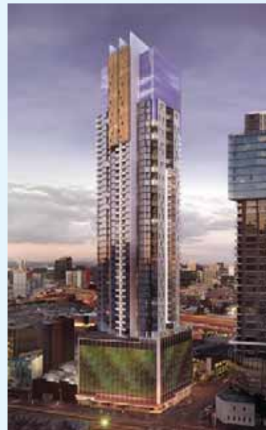
Platinum Tower, Southbank Victoria
